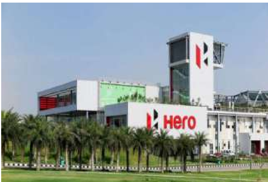
Green Factory Hero Motocorp, Rajasthan
